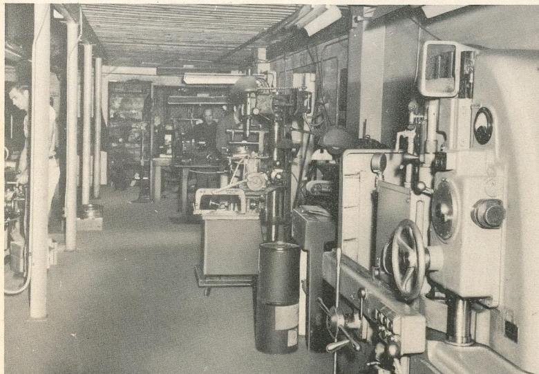
Maintenance shop showing Blanchard grinders, etc. for maintenance of lap plates to high degree of flatness.
